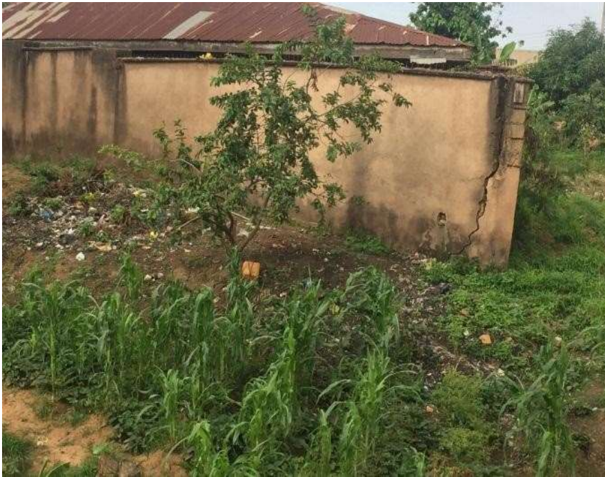
Plate 2. A building beside the open university at the verge of collapsing as a result of erosion
