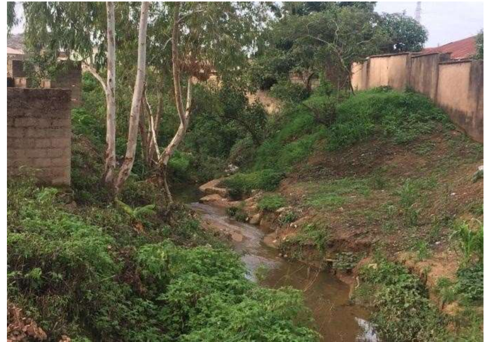
Plate 3. Buildings along a stream being threatened by erosion
