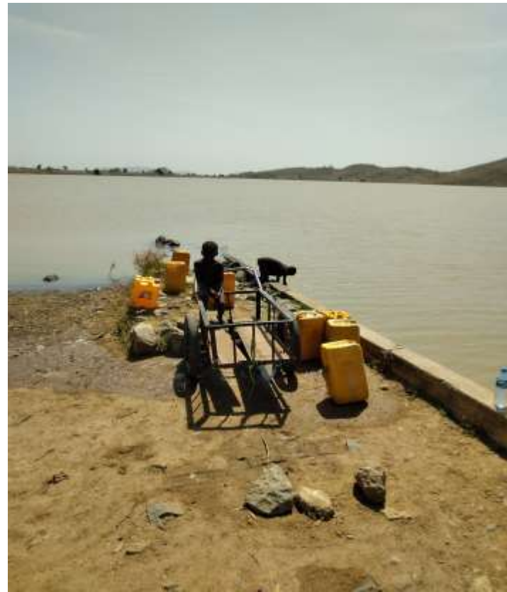
Plate IV: The Langtang Dam. The rhyolite hills at flank
