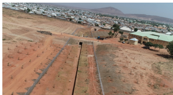
Before and after construction images of FCE (T) gully site in Gombe
