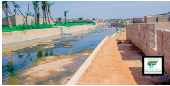
Flood control intervention at Jibia Town, Katsina State
