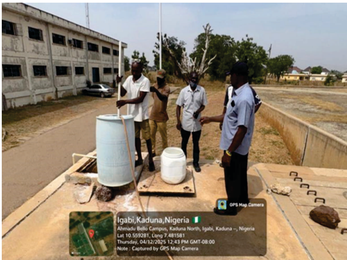
The manual method of applying chemicals for the water treatment
