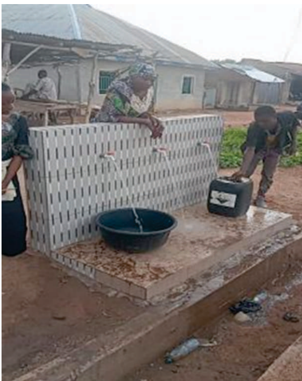
Borehole installed in Alapa, Kwara State
