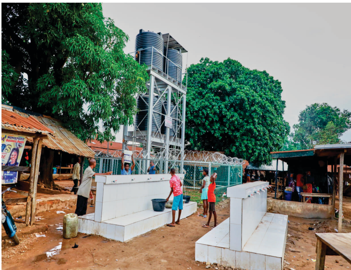
Solar Power Borehole in Kogi State
