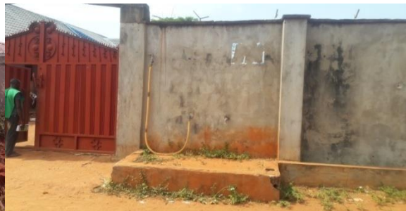
Private Un-functional Borehole
