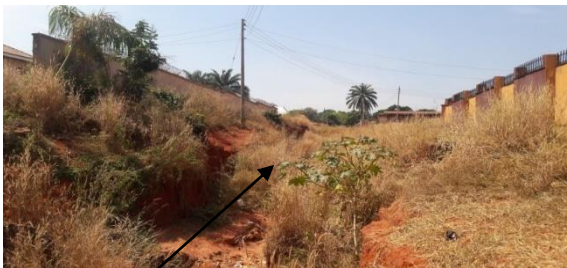
Road Leading to Area1 Eneokpoli Junction
