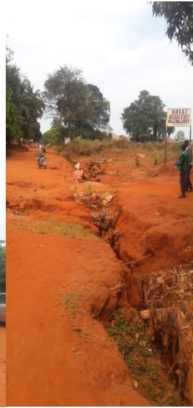
Road leading to Ogaji
