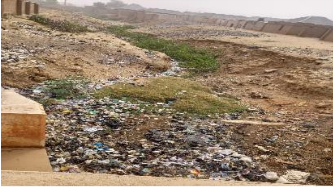
Plate 2. 3: A view of erosion gully site in Hamadu-Keffi in Akko L.G.A, Source: RAP Survey 2024.
