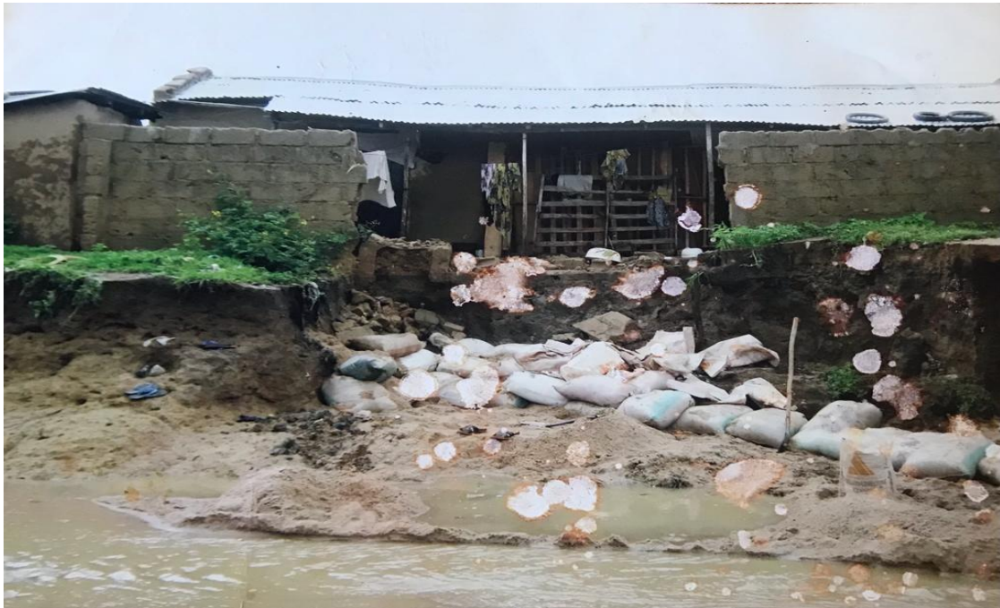
Plate 4. 2: Showing a structure being protected with sandbags at risk due to its proximity to the Gully.
