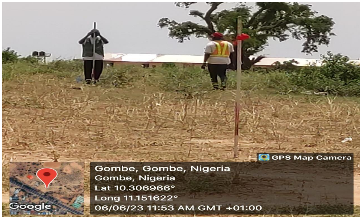
Plate 3. 4: Slope measurement at FCE Erosion Site.
