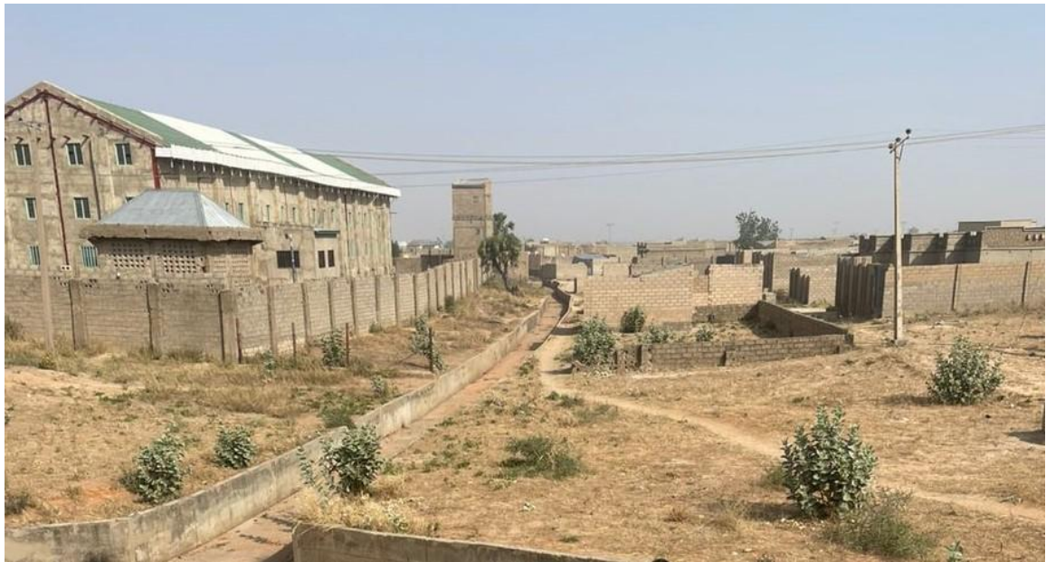
Plate 3-3: Structures at the beginning of the drainage canal
