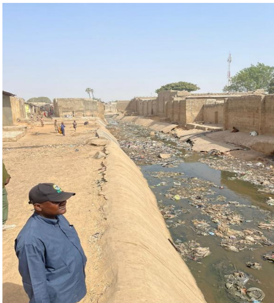
Plate 3-1 Section of The Drainage Canal
