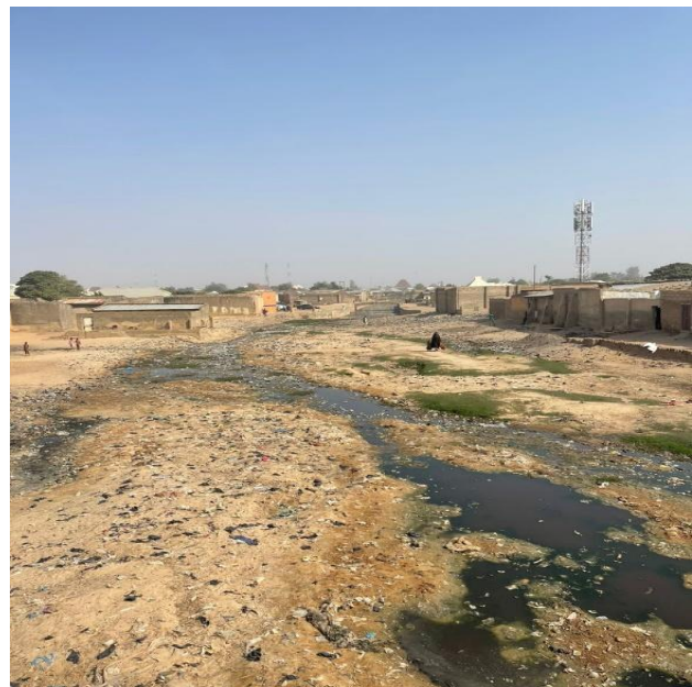
Plate 3-2: Section Of Washed Off Canal.
