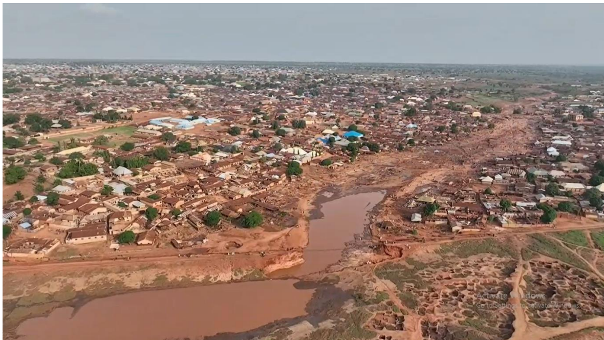
Figure 1.5: Environmental and Social Destructions by the Flash Flood in Mokwa
