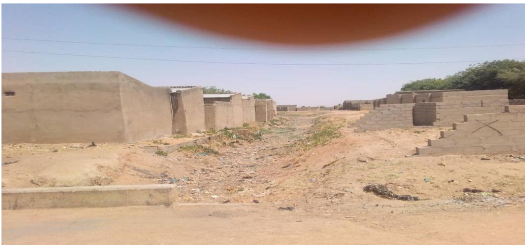
Plate 4.3: Structures Along The Drainage Canal
